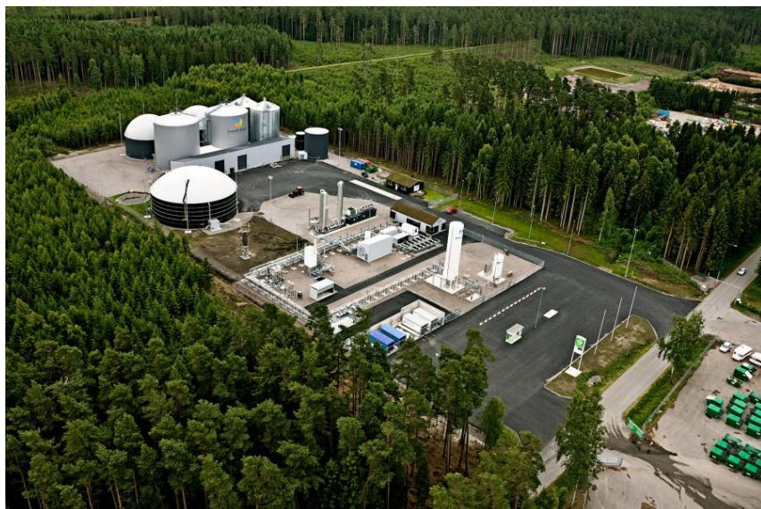
Lidköping Biogas: one of the world's first plants for liquefied biogas, as to fuel cars and trucks more
